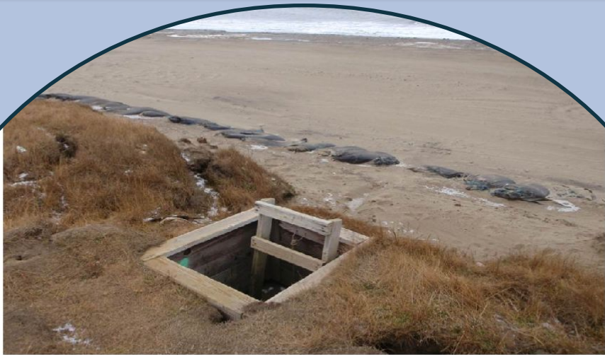
Food Storage Earthen Ice cellars (permafrost, rain, ice and snow for cooling)
